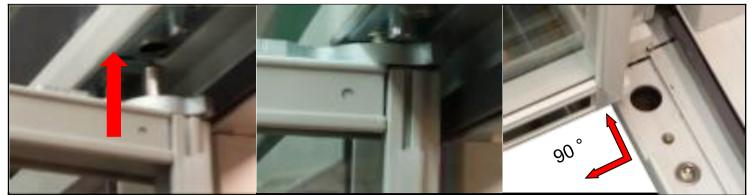
Hang in the doors - The bottom of the frame does not need to be fixed at this stage
