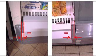
Distribute the gap between adapters and sidewalls identically on both side
