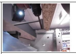
Depending on the fridge it may be necessary to drill a 7 mm hole in the upper console.
