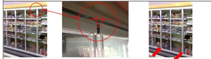
If the doors are not aligned in the internal/external direction, push slightly one corner of the frame in and pull the other corner out
