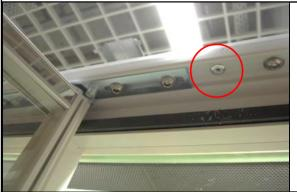
Fix the upper part of the frame to the adapter with 3<br/>rivets in the existing holes previewed in the frame.Ma<br/>rive<br/>use Alu Rivets Ø4,8x25 on the left and right and in the<br/>middle an Alu Rivet Ø4,8x10.Ma<br/>rive<br/>to a rive<br/>to a
