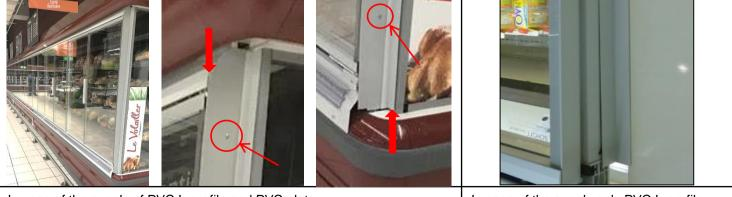
In case of the supply of PVC L-profile and PVC plate: 1- Install the PVC plate flush with the front of the frame to hide the profile and rivet it in the vertical bar of the frame. 2- Tape the L-profile in the angle between the PVC plate and the side wall In case of the supply only PVC L-profile: Tape the L-profile in the angle between the PVC plate and the side wall
